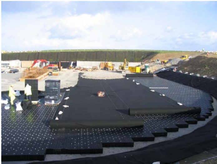
Figure 1. Constructing the geo-cellular runoff storage cell at Jersey Airport FTG.
